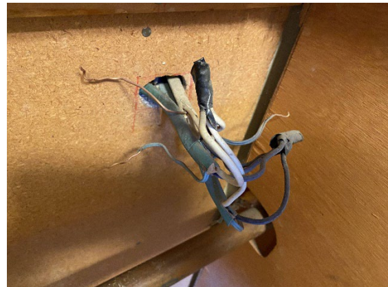
Figure 3: Two examples of exposed wiring in a home. Check all areas of a residence carefully to ensure there are no exposed wires. NEVER touch exposed wires.
