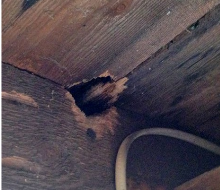
Figure 12: Rodent hole gnawed through a wood board
