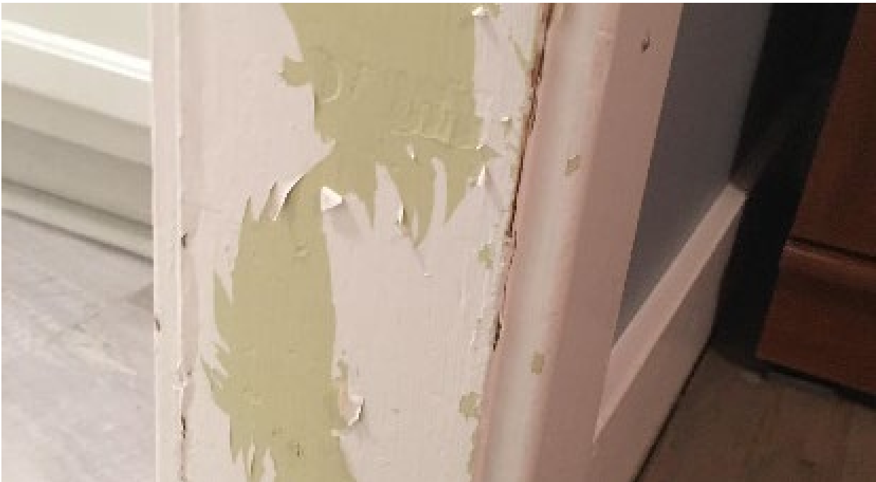
Figure 2: If paint is peeling back to reveal previous layers, especially in an older residence, pay close attention to the layers underneath, which may contain lead paint that has been painted over.
