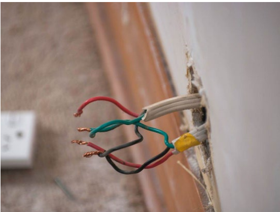
Figure 3: Two examples of exposed wiring in a home. Check all areas of a residence carefully to ensure there are no exposed wires. NEVER touch exposed wires.
