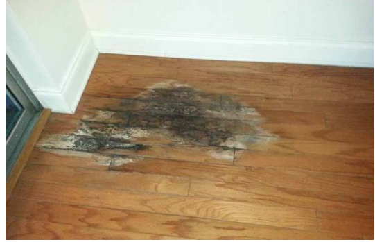
Water damage in wooden floorboards.
