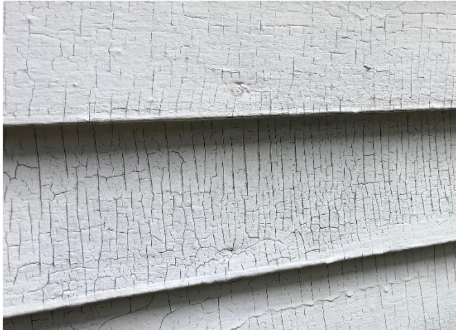
Figure 2: "Alligatoring" lead paint. This distinct pattern is a result of the oil base in lead paint. Not all oil-based paints are lead paints, but alligatoring is good indicator of lead paint in a residence.
