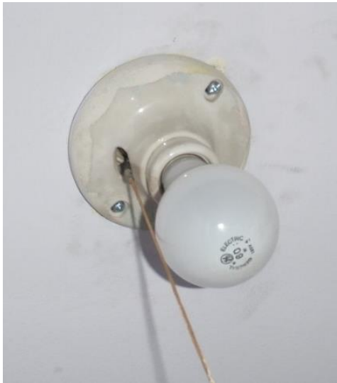
Example of an exposed incandescent lightbulb. Any kind of exposed bulb in a closet, basement, or garage is a safety hazard and should be replaced.
