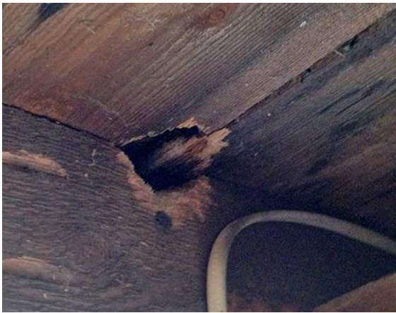
Rodent hole gnawed through a wood board
