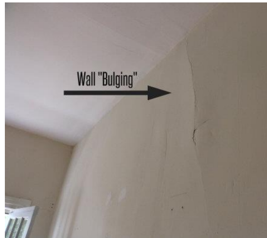
Bulging drywall is not always caused by structural damage, but when paired with other signs, it is a likely indicator.
