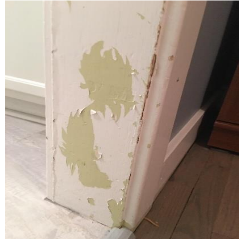
Figure 3: If paint is peeling back to reveal previous layers, especially in an older residence, pay close attention to the layers underneath, they may be lead paint that has been painted over.
