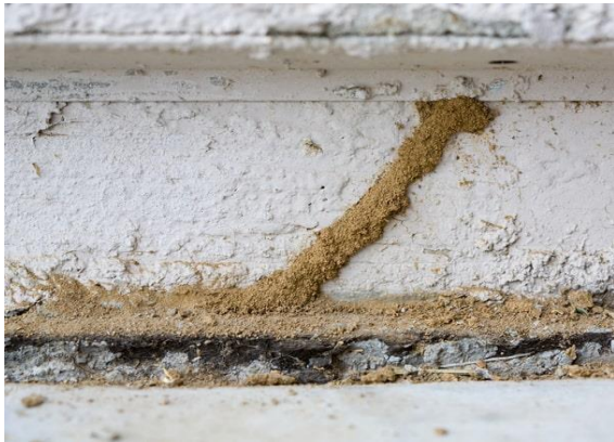
Termite tubes on the side of a house
