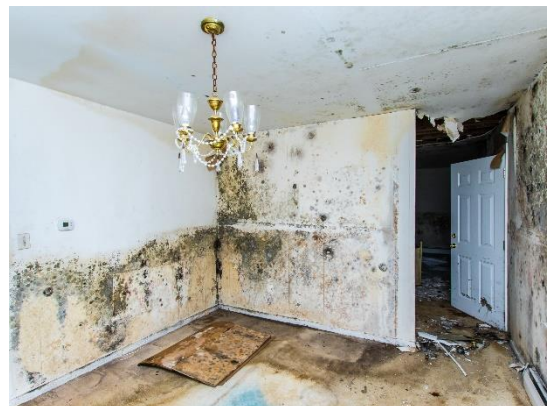
Mold on the walls of a house.
