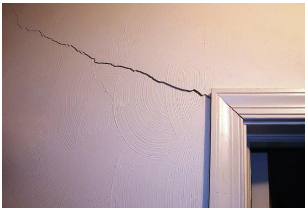
A large crack above a doorway. The presence of multiple cracks of this size is very concerning and a likely sign of structural damage.
