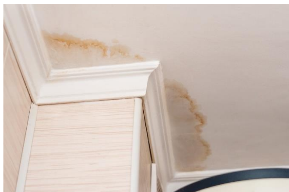
Water stains in a ceiling.
