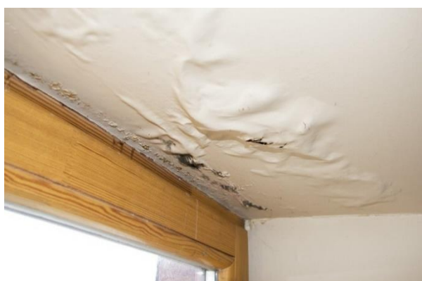
Bubbling paint caused by water damage.
